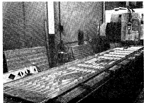
Fig. 13 Numerically controlled machining of an upper wing skin panel.
